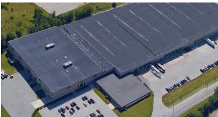
Barrie, ON (CAN) - High Performance Doors
